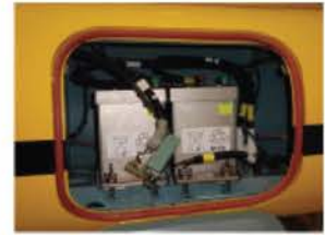
EC130 SECOND BATTERY INSTALLATION
